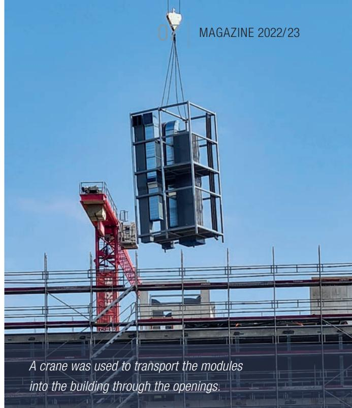
*A crane was used to transport the modules into the building through the openings.*
